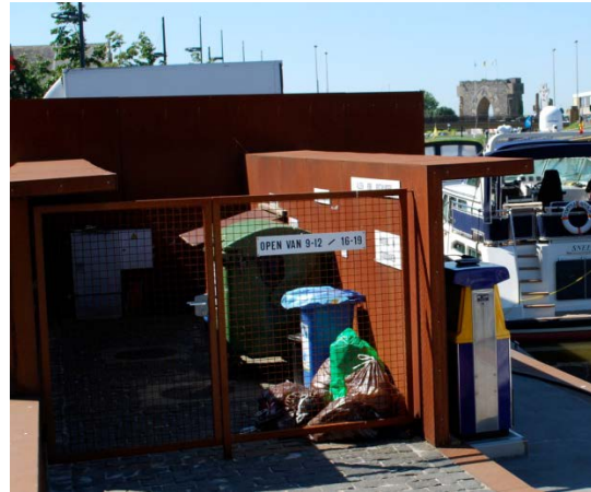
Combined reception facility for bilge water and garbage in a marina in Belgium (Photo credits: Peter Van den dries)
