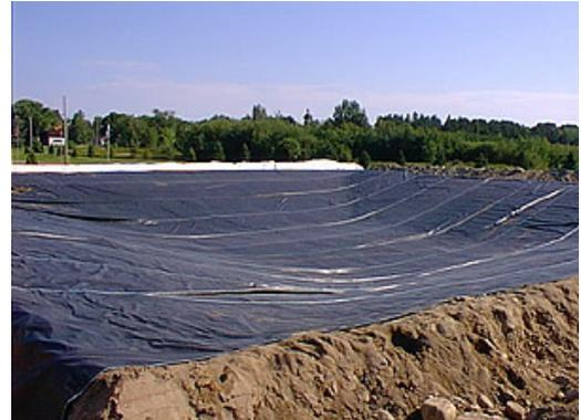
Dewatering is the result of physical separation according to the specific weight and evaporation of liquids (during a longer period). Removal of free liquids from the lagoon can easily be achieved with pumping from the surface while sediments can be removed by dredging or digging. Cleaning of the lagoons (sediment removal) is required in regular intervals.
