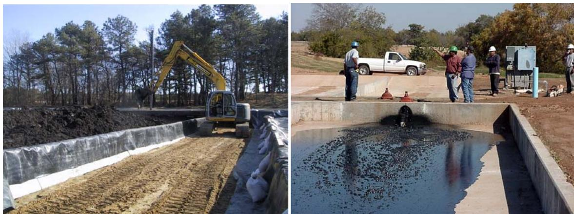
Drying beds are not particularly suitable for oily sludge's, as drying and draining are slow and the drain might be clogged with oil.
